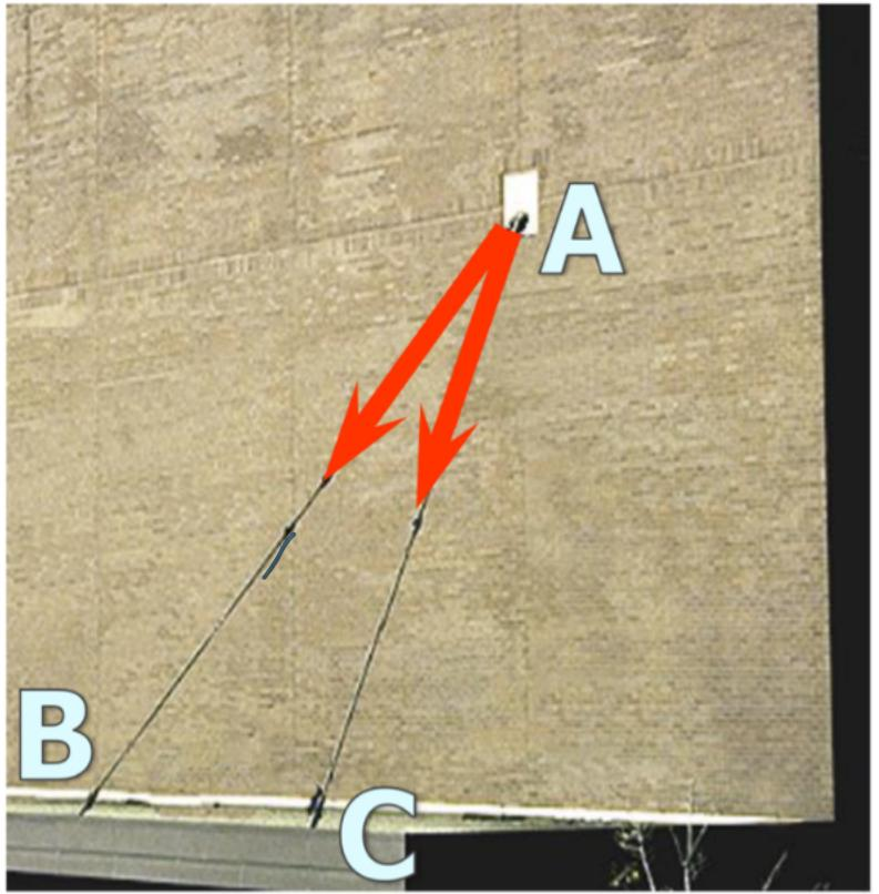
The roof is supported as shown. If the cables exert forces of  $F_{AB} = 100 \text{ N}$  and  $F_{AC} = 120 \text{ N}$  on the wall hook at A, determine the magnitude of the resultant force acting at A.
